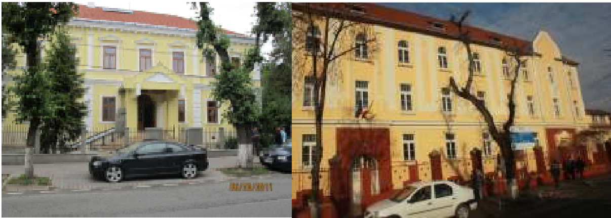
Rehabilitation – "Andrei Mureșanu" National College of Bistrița
